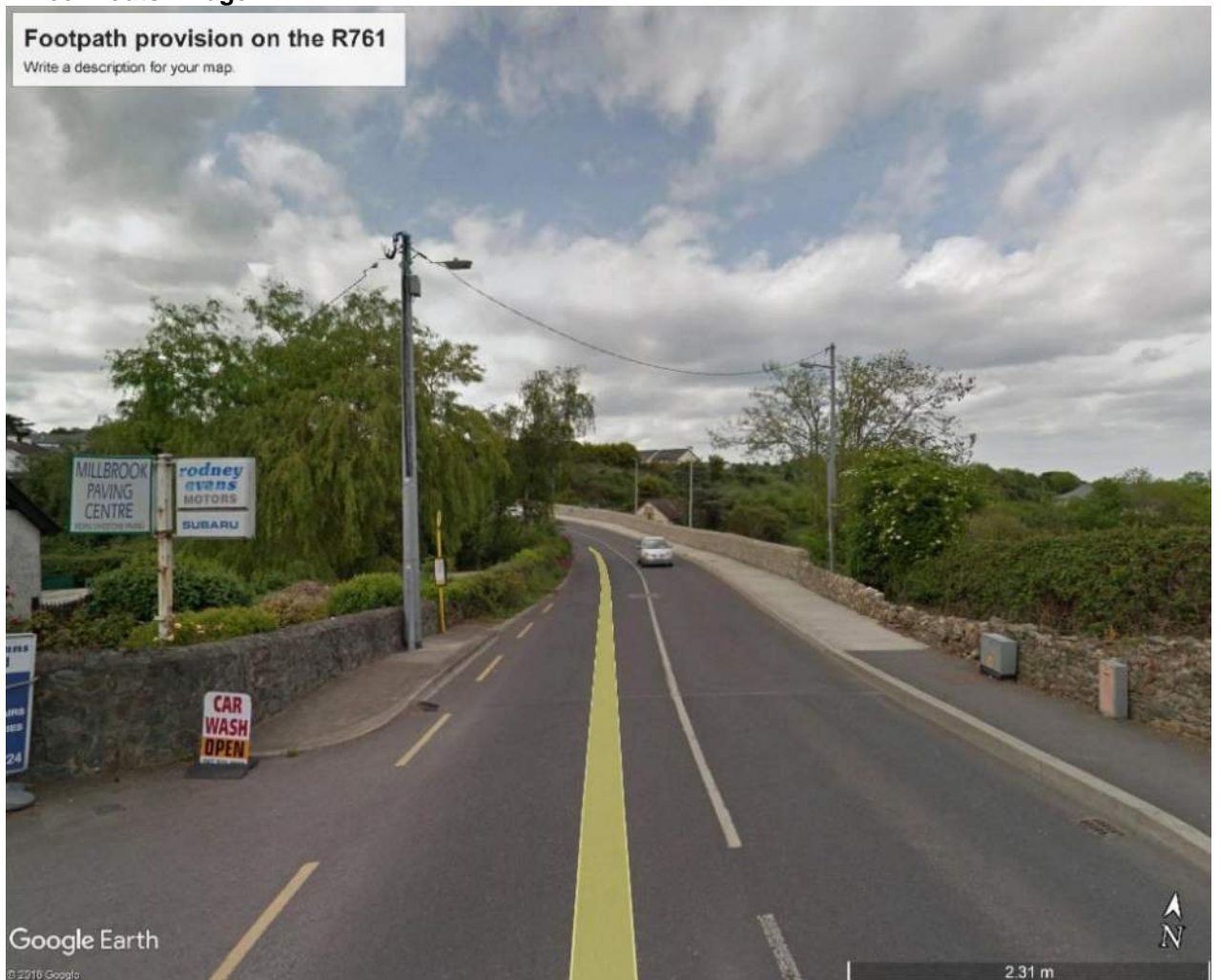
Figure 3 – Kilcoole Road - end of the footpath provision on the western side of the road approaching Three Trouts Bridge
