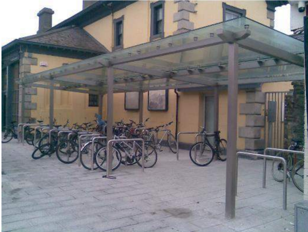
Figure 6 – Cycle Parking at Greystones Railway Station
